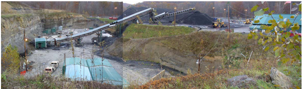
View of Sago mine portals to the left and the “hill” to the right with bathhouse and offices at far right.
